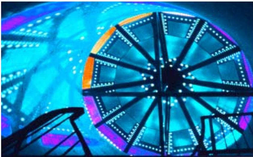
▲ **TOWER OF THE ECLIPTIC**, SWANSEA, WALES. HAND-BLOWN GLASS, DICHRONIC FILTERS AND DRILLED ALUMINIUM. FIVE-METRE DIAMETER ROOF LIGHT TO ACCESS TOWER. ARCHITECT: ROBIN CAMPBELL
